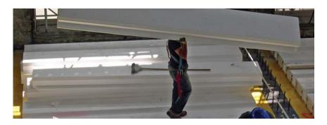
Compared to a floor in clay/concrete mix or to plates, with the same thickness, the weight is cut about 100 kg per m2. This means a consistent saving of iron, concrete and labour.
