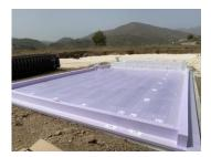
As for our foundation insulation we use an EPS (Expanded PolyStyrene) based system. It consists of loose bottom plates and side walls, which are provided with unbreakable strips as reinforcement. That makes this system the strongest in the market. In addition, this system is significant easier and faster to process than traditional systems. For example, additional sand or the use of separate corner pieces are not necessary. A three-part system also creates much less waste.
