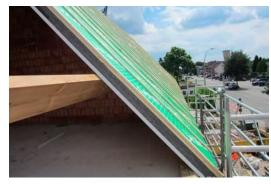
Insulating your roof properly means a lower U-value and build airtight without thermal bridges. The way to do this is insulate from the outside using self-supporting insulating sandwich elements which have the property to make very effective use of the insulation.
