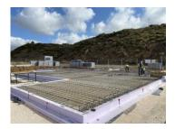
Eco Building Group uses an insulating formwork that ensures a strong connection to the walls without thermal bridges.
