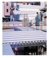
Panels are originally self-standing, that is they can stand any weight (concrete casting, workers, reinforcement steel, etc.) with traditional and simple shoring system with prop supports at a maximum distance up to 2 meters.
