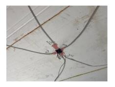
The electric cables are laid into a melted space into the internal insulation with a special hot knife saving the customer costs and time of intensive break works.
